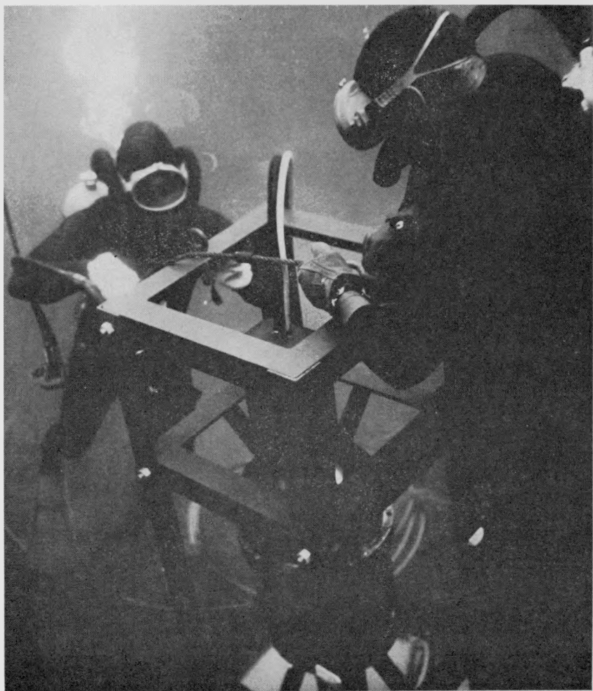
One of Two Special Nuclear-Powered SNAP-21 thermoelectric generators, suspended in a support frame, is shown being maneuvered into place by Navy frogmen on the ocean floor about 150 feet under the surface off San Clemente Island, near Long Beach, Calif. The frame will keep the unit about 5 feet above the floor during an extended testing period. Ocean testing of three such 10-watt units, fabricated by the Minnesota Mining and Manufacturing (3M) Co., St. Paul, Minn., began in June 1969.
