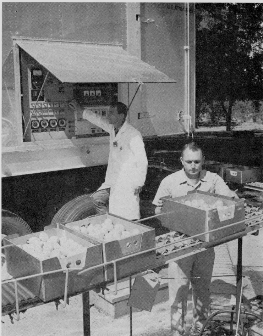
One of the Mobile Irradiators in operation for AEC studies on irradiation processing of foods to prolong the storage life is shown as technicians prepare to irradiate lemons at the University of California's Davis Campus. This irradiator is mounted on a truck for easy movement between crop harvests.
