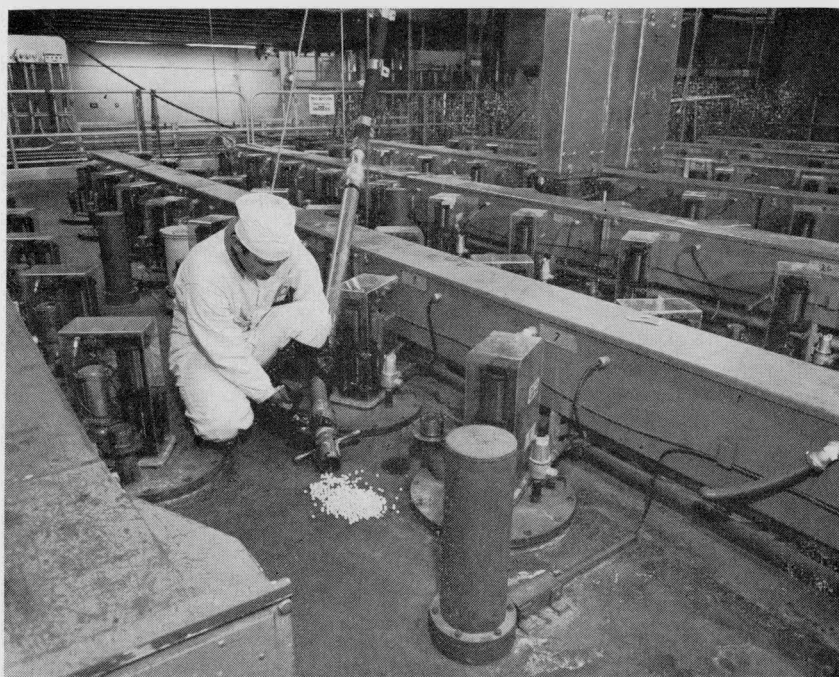
The Ball Safety System provides Hanford's "N" reactor with an emergency shutdown capability independent of the reactor's horizontal control rods. The control elements for this system are the small samarium oxide balls shown in front of the operator. Hoppers, each holding 108 balls, are embedded in the biological shield on top of the reactor, each one over a vertical channel through the reactor. The hopper gates, held closed by battery-powered solenoids, are designed to open if any number of "out-of-limits" events occur, pouring the neutron-absorbing balls into the reactor. They absorb so many neutrons that the chain reaction is stopped and the reactor shuts down.
