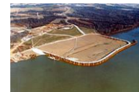
Above: Cofferdam on Ohio River Below: Reinforced Concrete Base
