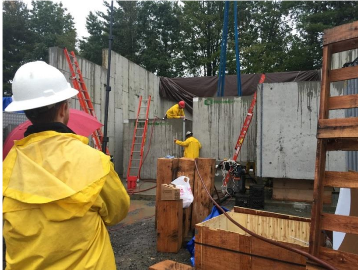
Figure 6 - Modules placed into position
