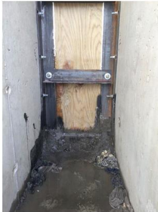
Photo 4 – Leaking at Bulkhead (Left side looking upstream).
