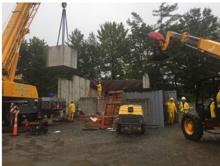
Figure 5 - Modules placed into position
