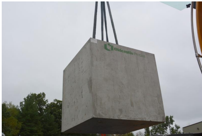
Figure 4 - Module hoisted into position
