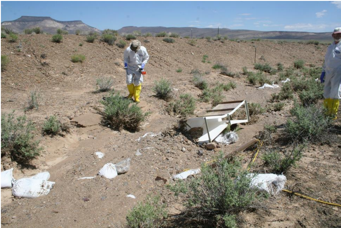
Figure 6. Flume moved downstream approximately five or six feet after the July 28, 2013, storm event.
