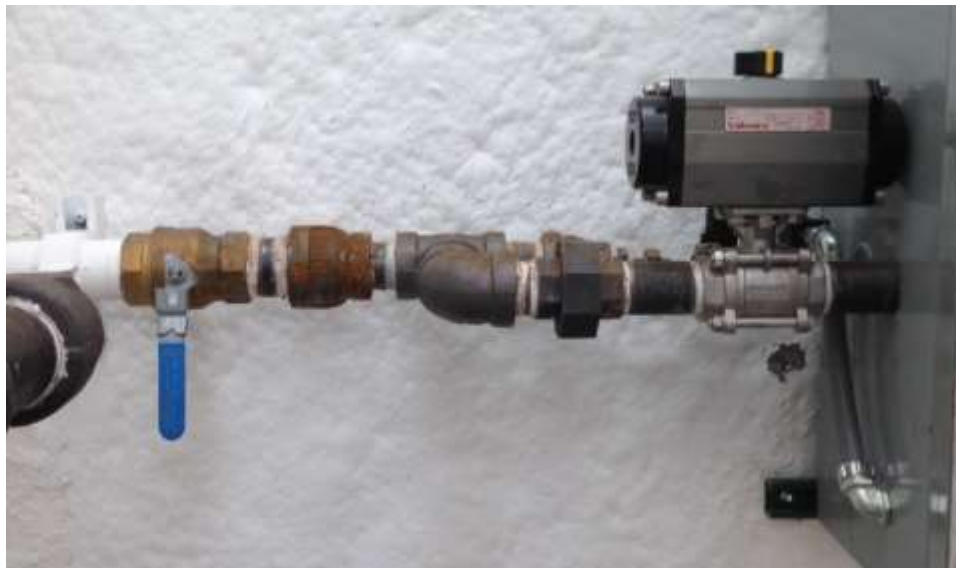
Figure 57. Control Box Entry (2" pipe to 1 1/2" reduction)
