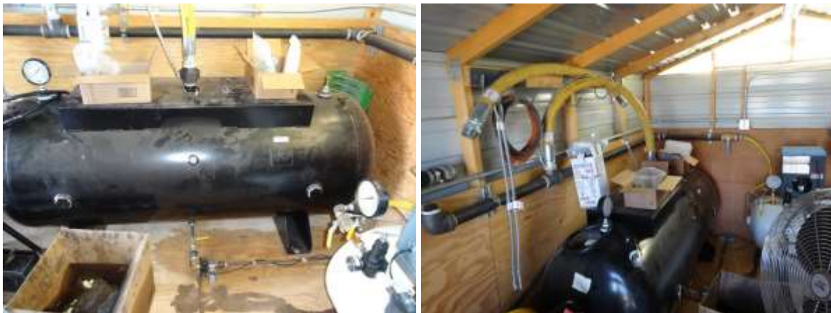
Figure 55. 240 gallon air receiver with auto drain and pressure relief valve
