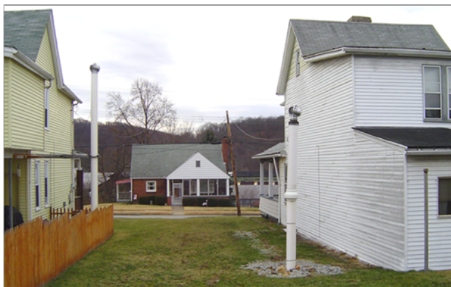
Figure 3: High CH 4 concentrations from leaking gas wells forced residents of these houses to live elsewhere for almost a month in 2003. Vertical white pipes are vents installed to draw CH 4 away from foundations.
