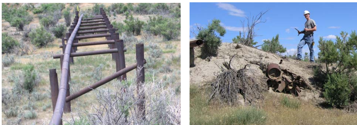
Figure 8: A pipeline bridge made from well casing and a pile of buried ferromagnetic trash created helicopter magnetic anomalies that resembled wells. Twenty four of 153 TMF anomalies were not visible wells; 93 of 224 CVG anomalies were not visible wells.
