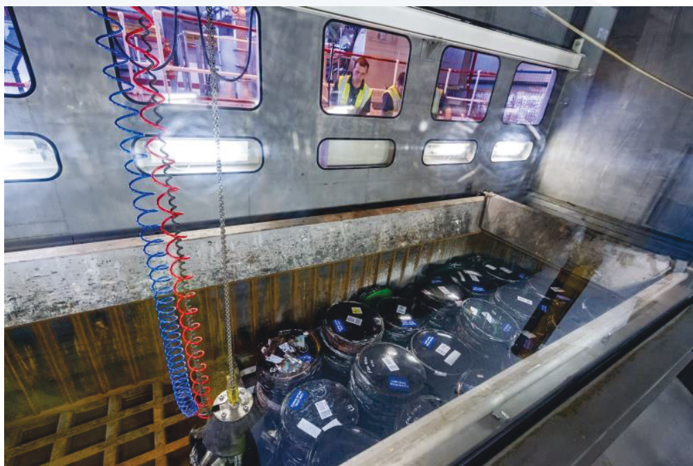
Figure 19. Photograph of an ISO-Freight Container in Dounreay's WRACS Facility with Super Compacted LLW Waste Drums Being Loaded (Ref 251).
