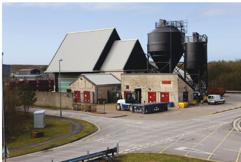
Figure 12. The LLWR Grouting Facility.
