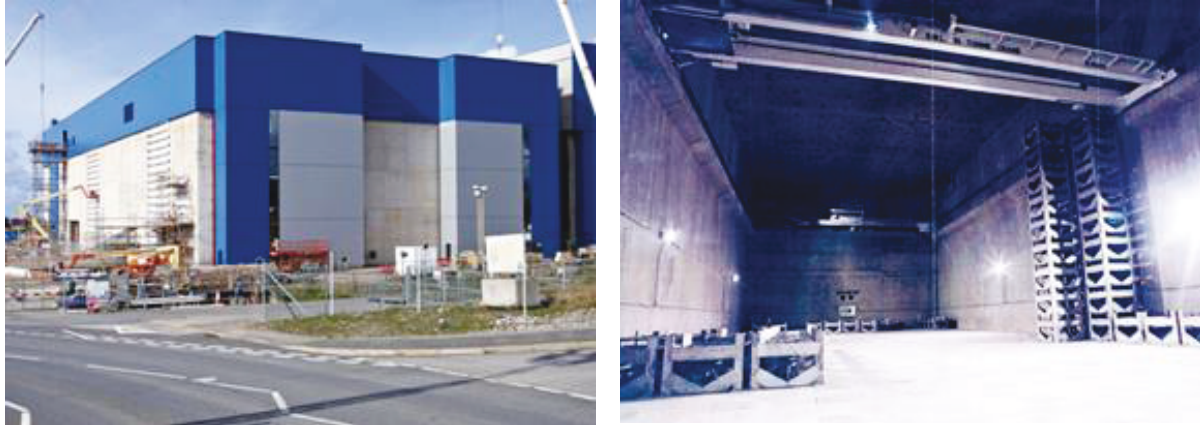
Figure 51. ILW above Ground Storage Facilities at Sellafield, Cumbria.
