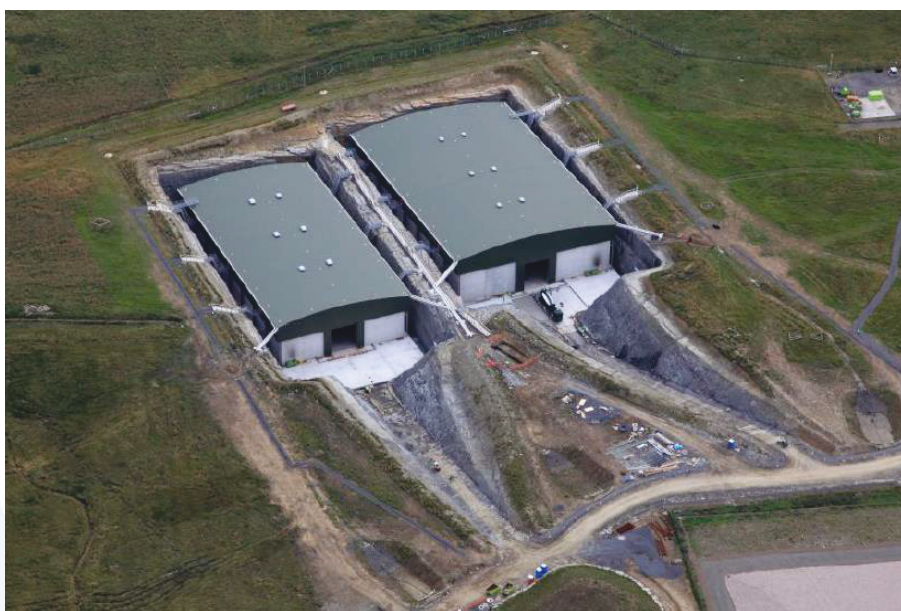
Figure 45. The Recently Constructed LLW Vaults at the Dounreay site (Ref 270).
