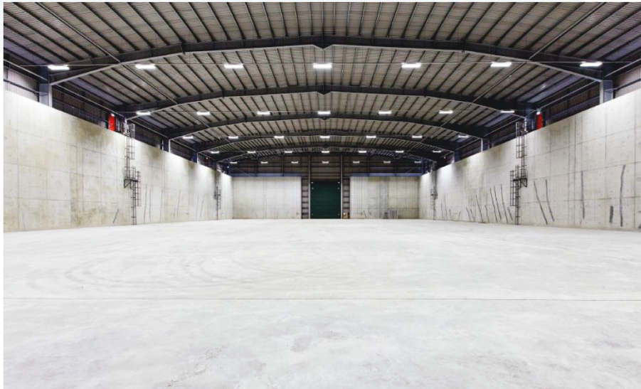
Figure 46. An Interior View of One of the Recently Completed Dounreay LLW Vaults, Post-Construction (Ref 270).
