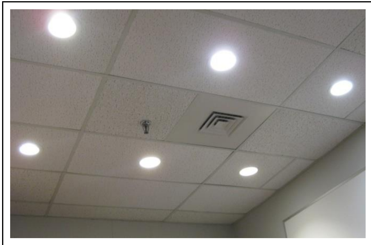
Figure 4D-1. Picture of the Downlights Used in the RTOL Test After Installation in a Ceiling in a Common Area in RTI Offices
