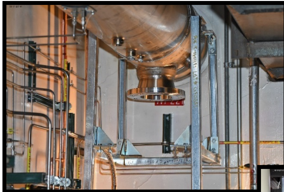
Exhaust Stack Showing Penetrations
