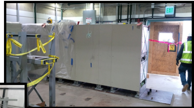
Battery Racks in Place
