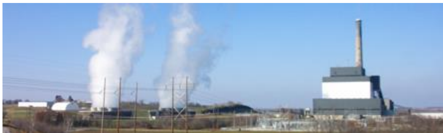
Figure 1. Ottumwa Generating Station
