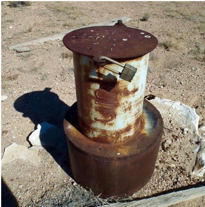
Figure 26. U-10L 1 wellhead (photo courtesy of NSTec, 2015).
