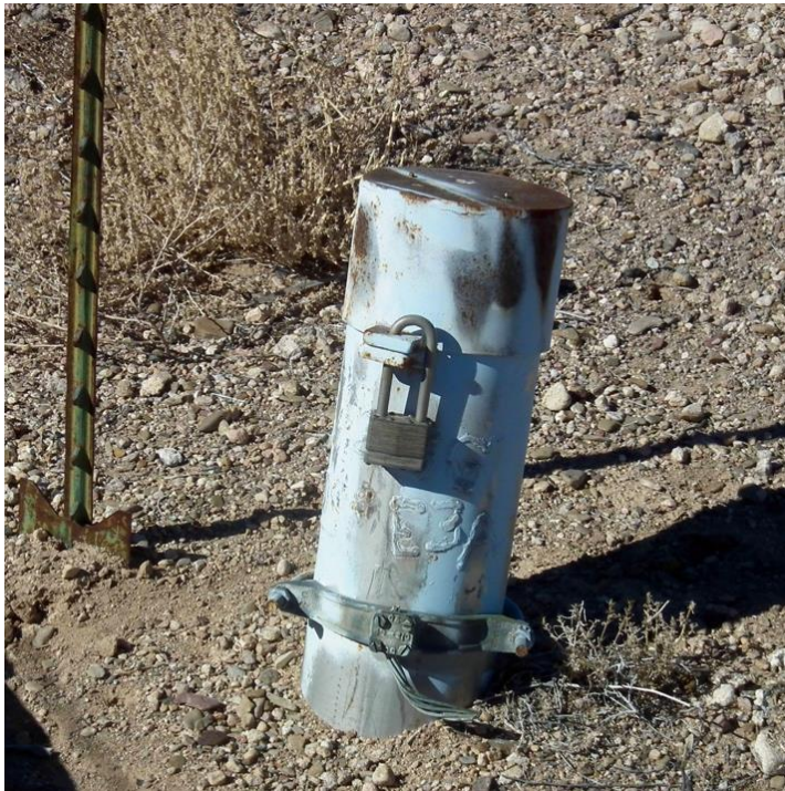
Figure 21. U-2gg PSE 3A wellhead (photo courtesy of NSTec, 2015).
