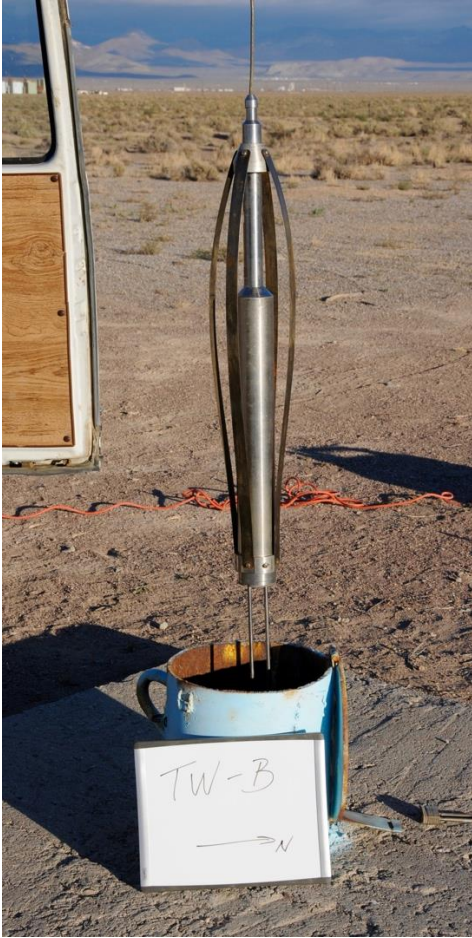
Figure 8. Photograph of video camera being lowered into TW-B.
