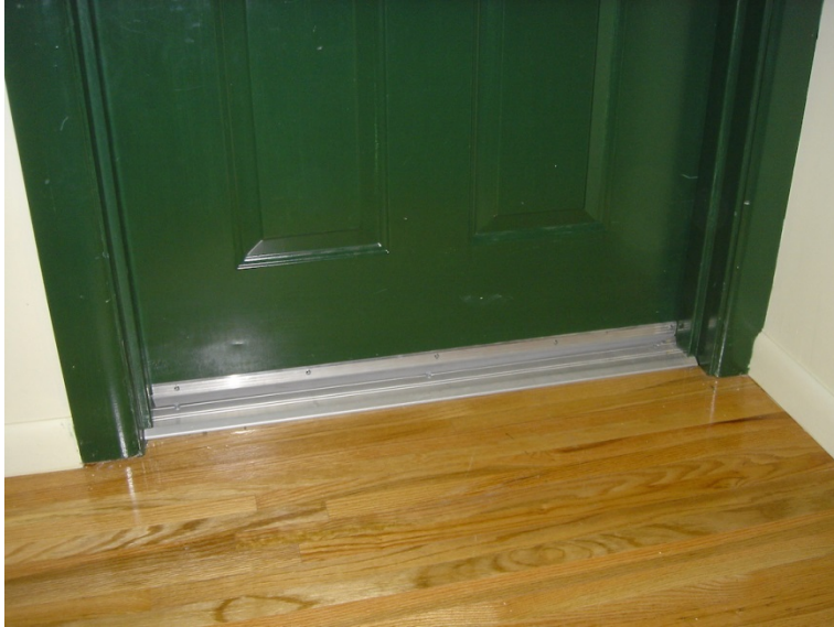
Figure 5. Weatherstripped corridor doors—Ventilation air is prohibited from being introduced into multifamily units from corridors; doors from multifamily units to corridors are typically weatherstripped
