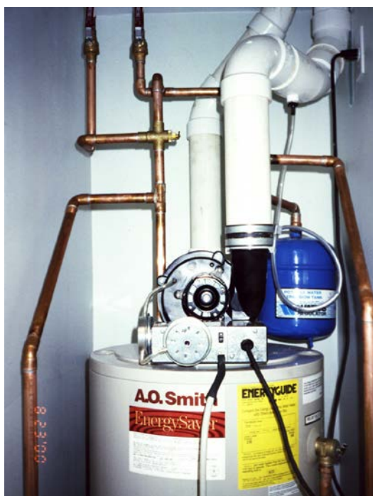
Figure 15. Gas water heater—Gas water heaters should be sealed combustion two-pipe systems vented directly to the exterior with combustion air ducted directly to the water heater
