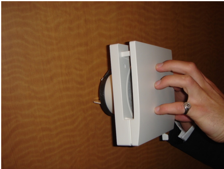
Figure 6. Passive air inlet—Ventilation air can only be introduced into multifamily units by infiltration through exterior walls or directly into the units by ducted supply or passive air inlets (holes in the exterior walls)
