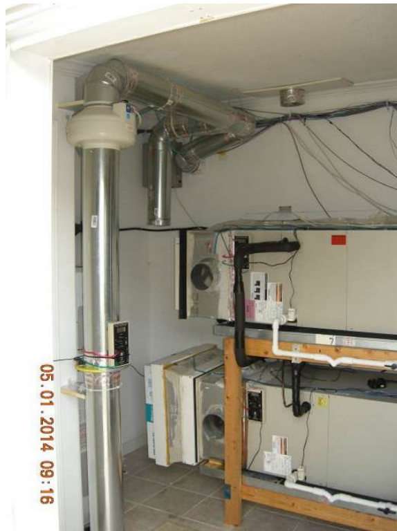
Figure 3. Mechanical ventilation OA is brought into the MH Lab using an in-line fan and measured with a calibrated iris damper. This photo shows the option that delivers the air near the return of the SEER 22 (top) and SEER 13 central systems.
