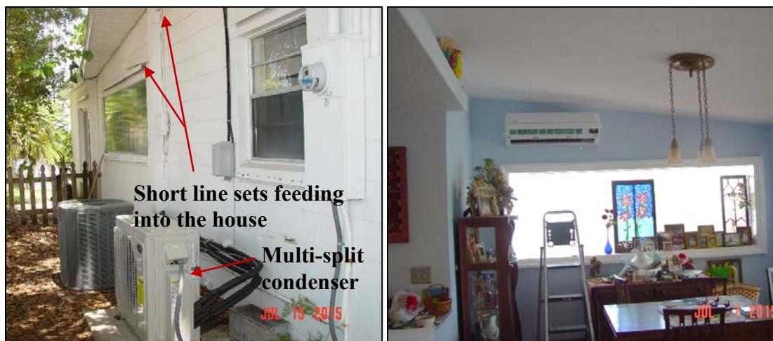
Figure 9. Condenser location, nearby electrical panel, and short exterior line set runs (left); centrally-located, wall-mounted fan coil (right)
