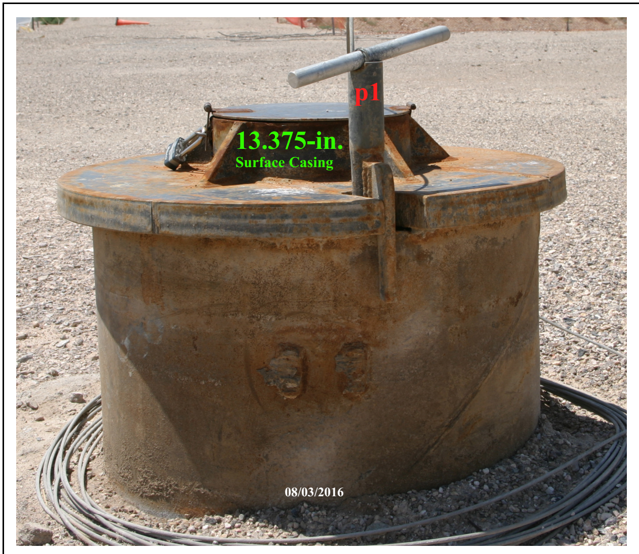
Figure 3-3 Photograph of Well ER-2-2 Wellhead
