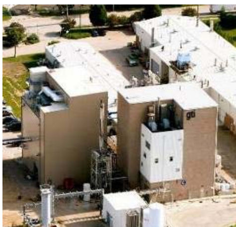
Figure 1. The pilot plant gasifier test program used existing equipment and infrastructure located in the Advanced Gasification Test Facility (left) and Flex Fuel Test Facility (center) at the Gas Technology Institute.
