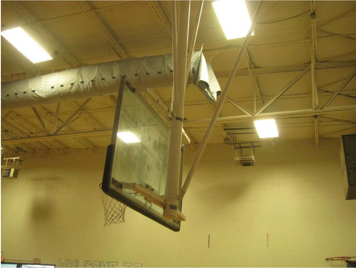
Photo 9 New Fabric Duct for Gymnasium
