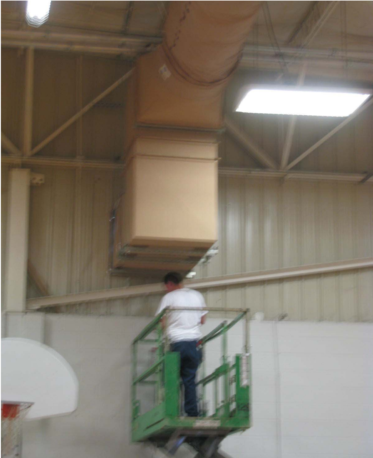
Photo 12 Ductwork for Gym
