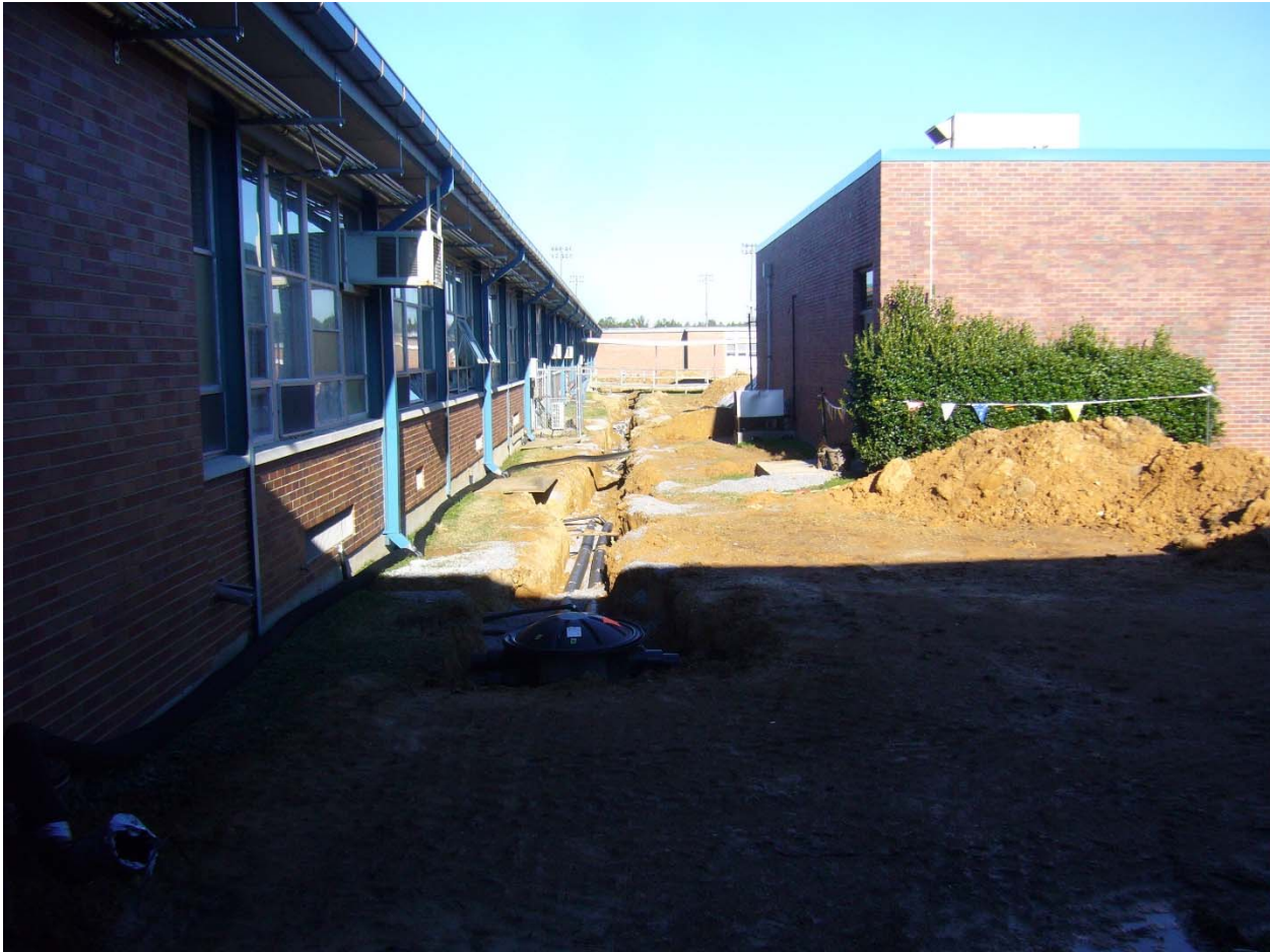
Photo 1 – Exterior Geothermal Main Distribution Loop
