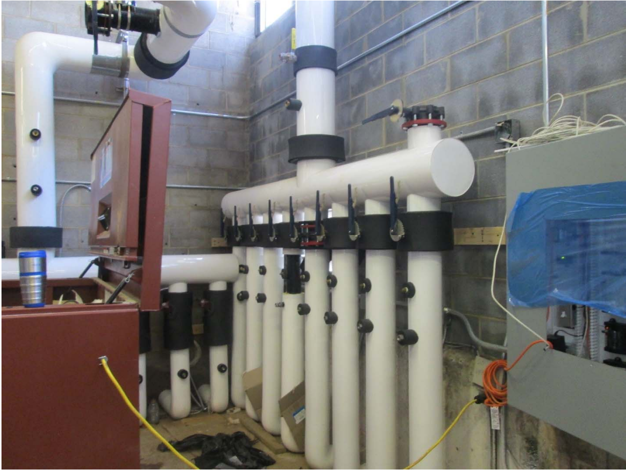
Photo 3 Geothermal Loop Header
