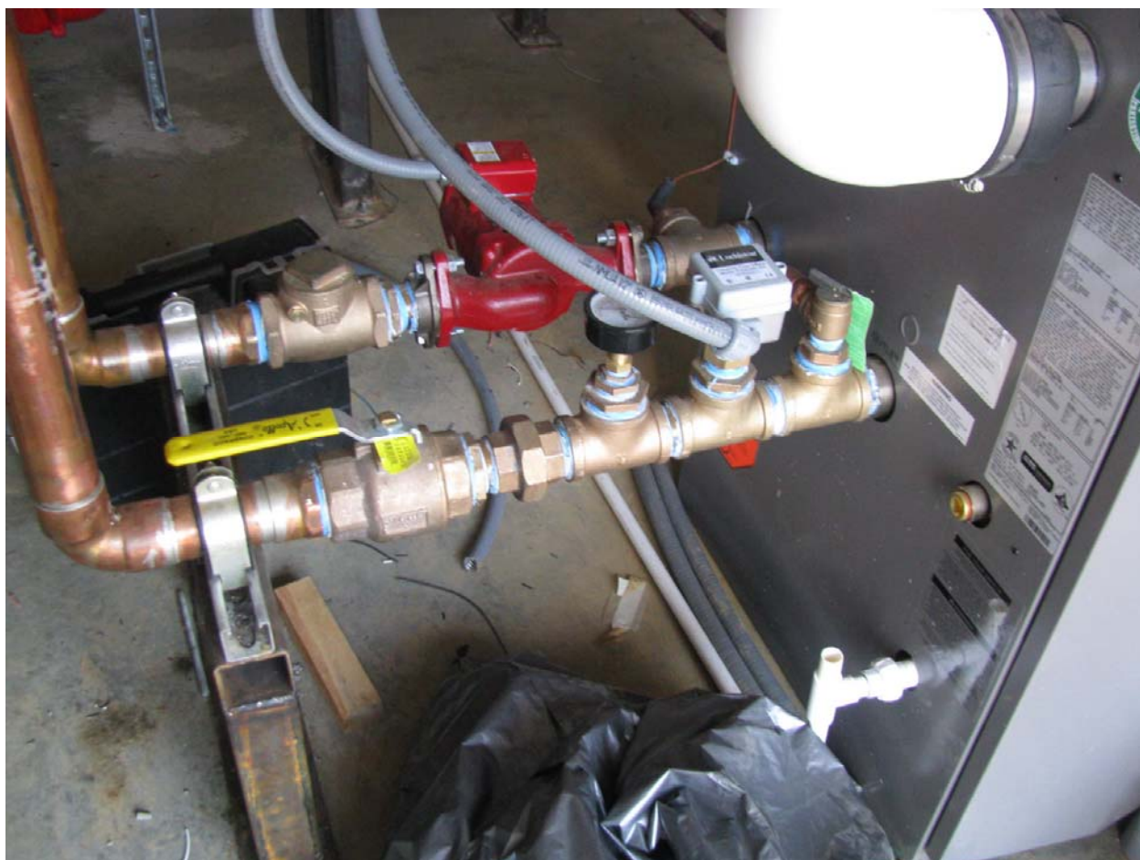
Photo 10 Typical Heat Pump Piping Connection
