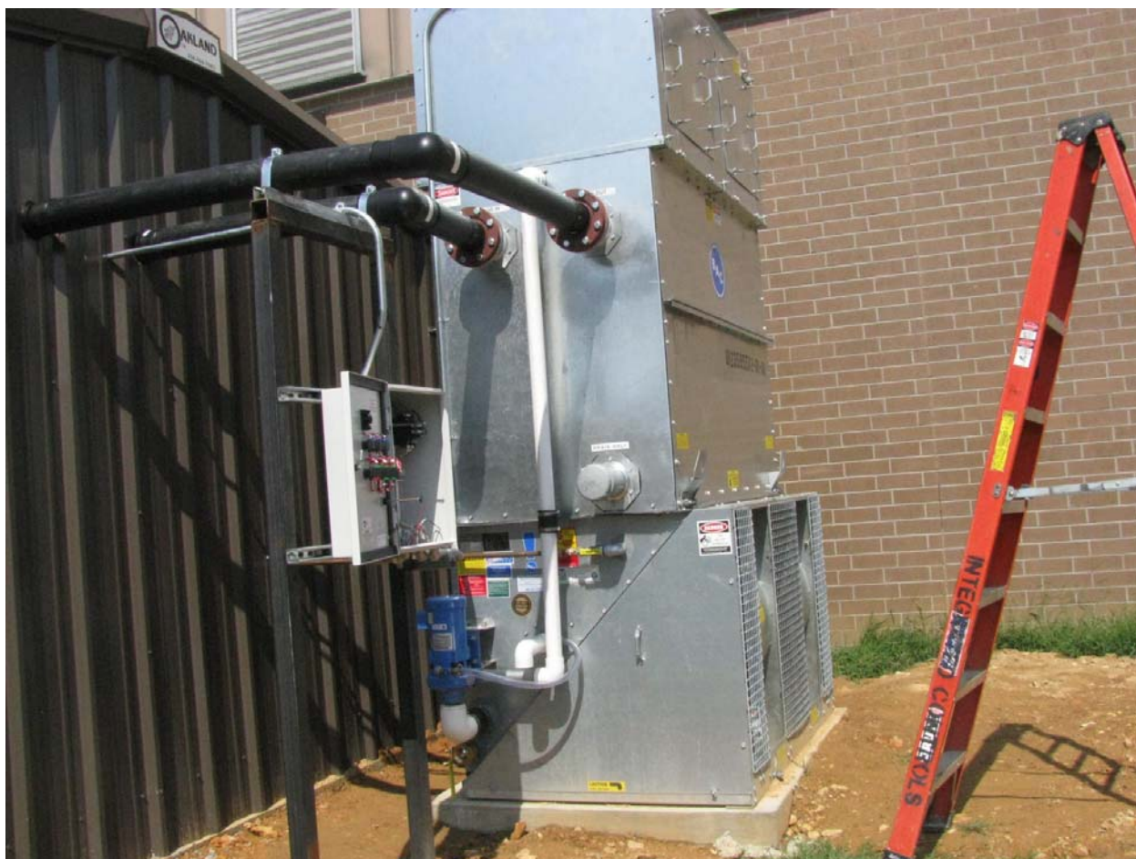
Photo 7 New Cooling Tower
