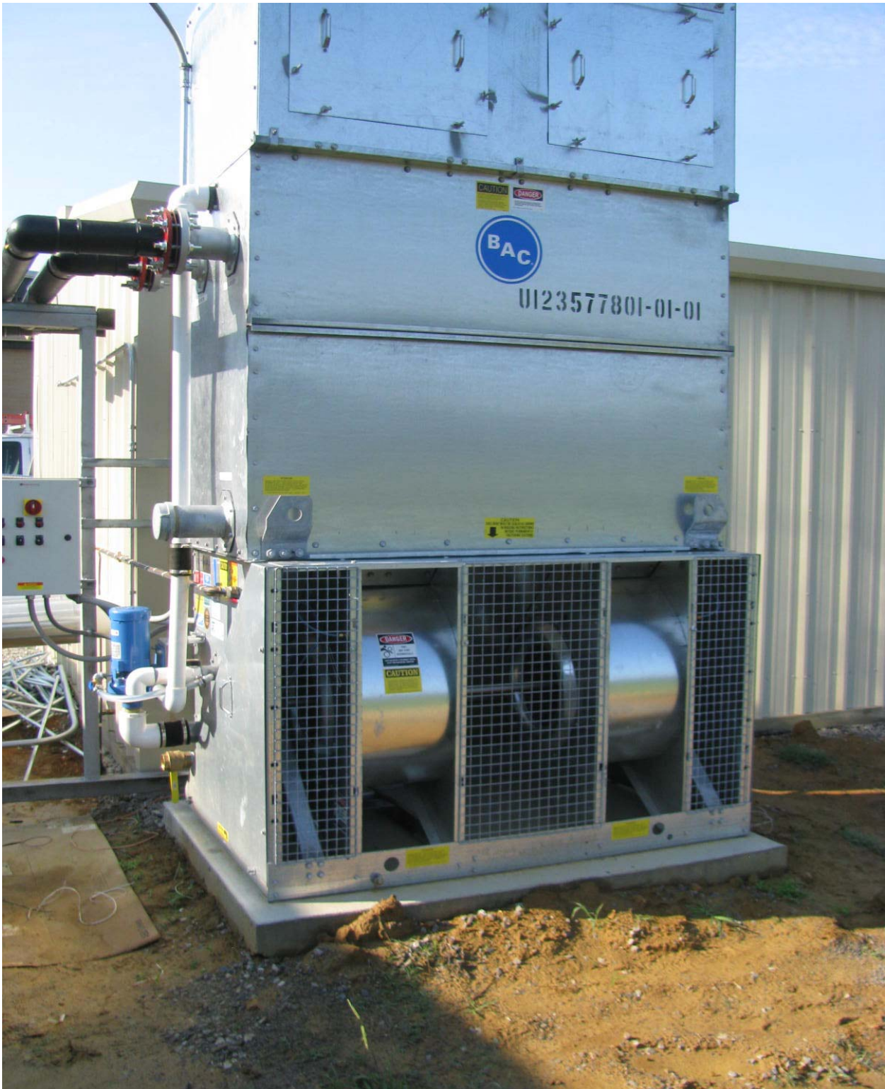
Photo 11 Cooling Tower for Gym & Locker Room/Weight Room
