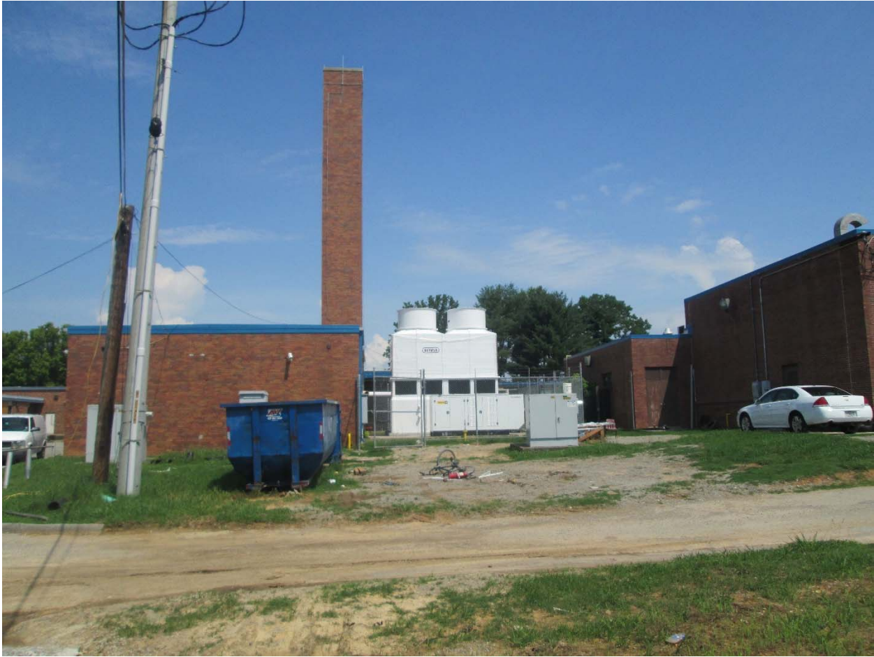
Photo 2 Cooling Towers for HY-GSHP System
