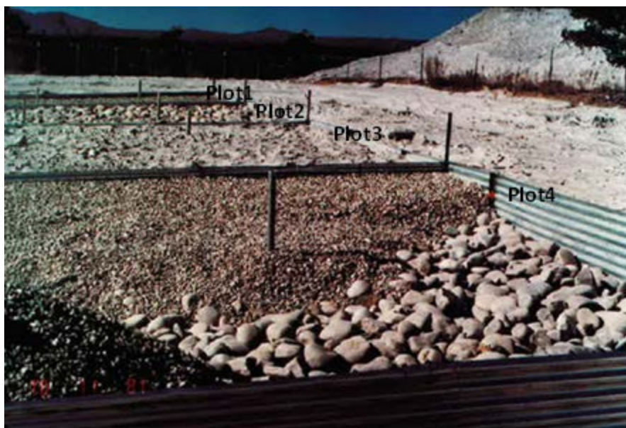
Figure 6-1 Four biointrusion-barrier test cover plots constructed along the north central border of Pit 25 in 1981. Portions of the barrier materials are shown here during construction, before the final 15 cm of topsoil was added on each plot.
