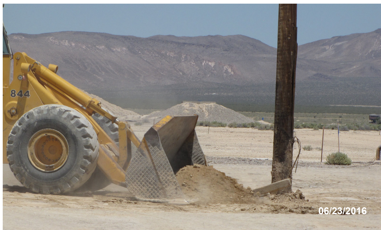
Figure 2-7 Removal of Hamilton Soil/Debris Pile
