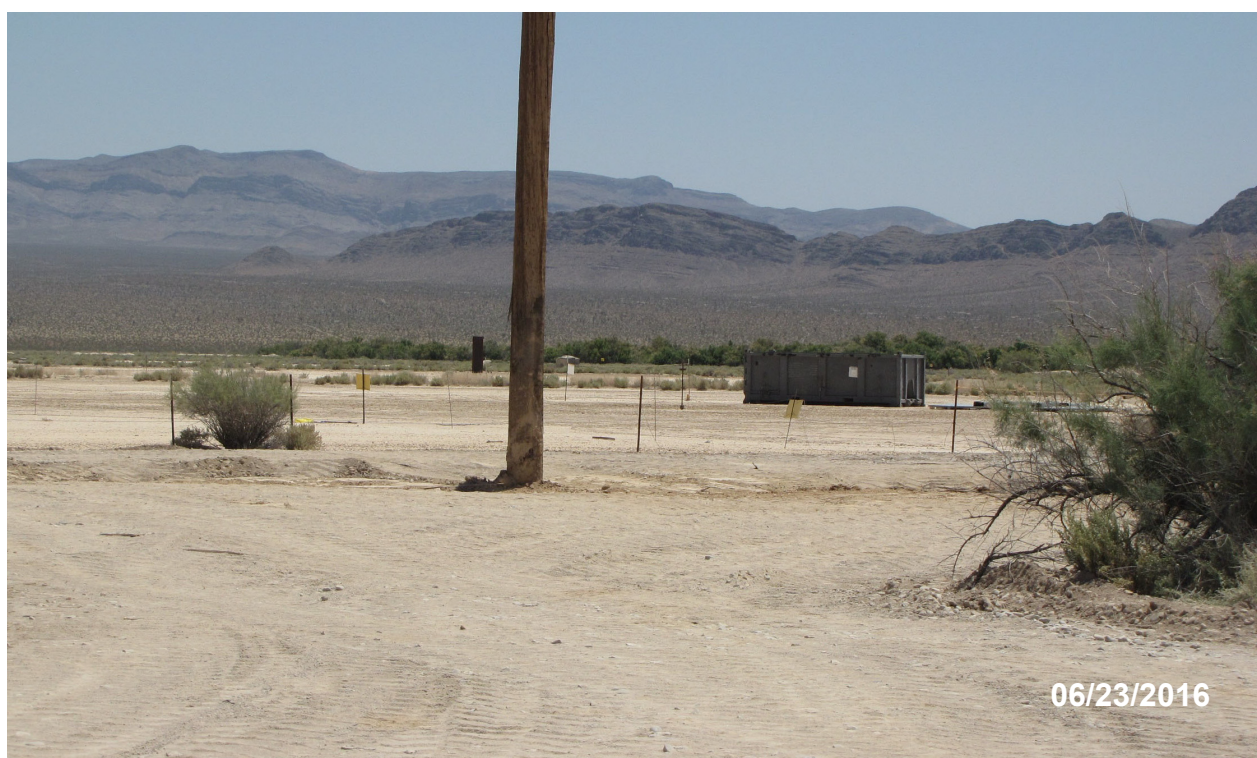
Figure 2-12 Hamilton Site after Removal of Soil/Debris Pile
