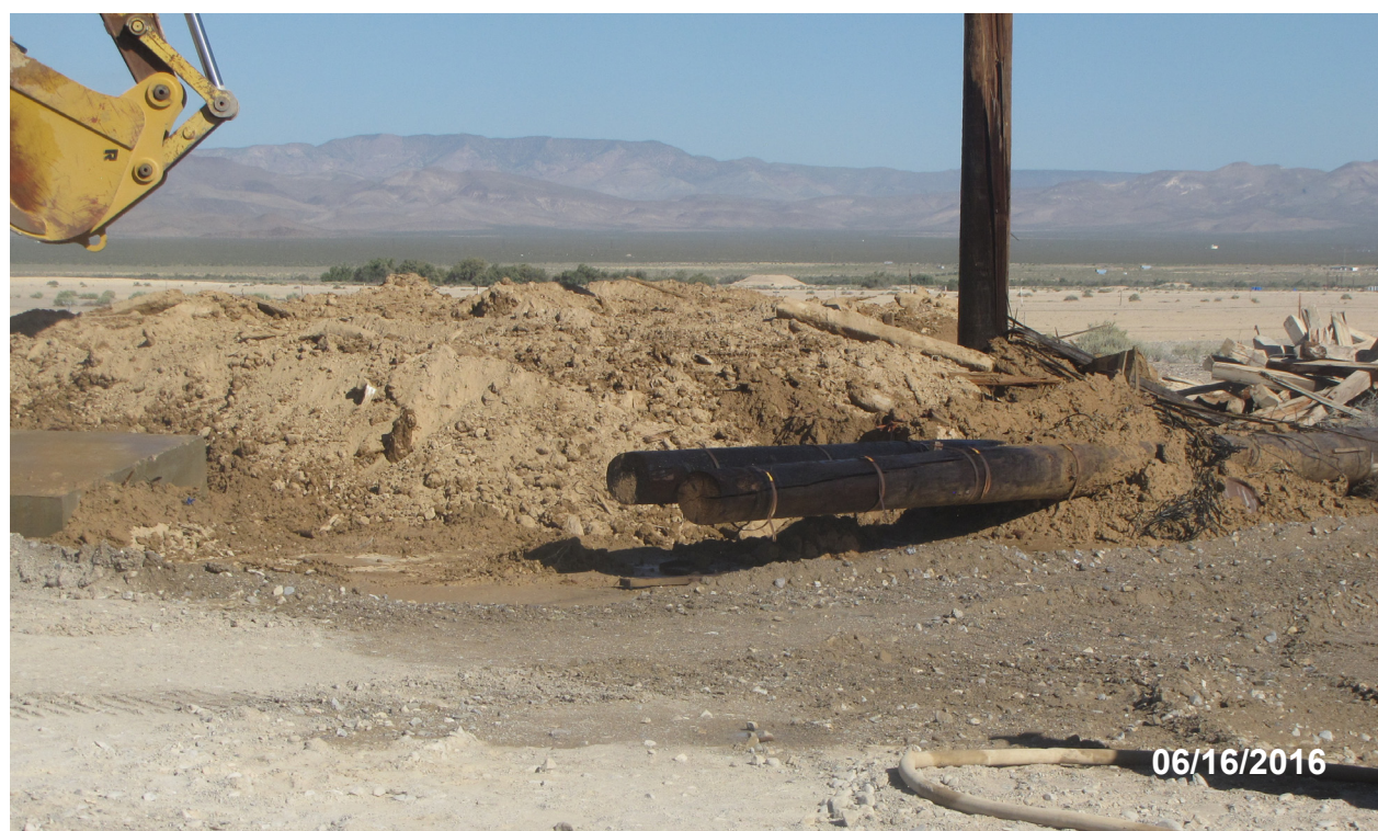
Figure 2-5 Removal of Hamilton Soil/Debris Pile
