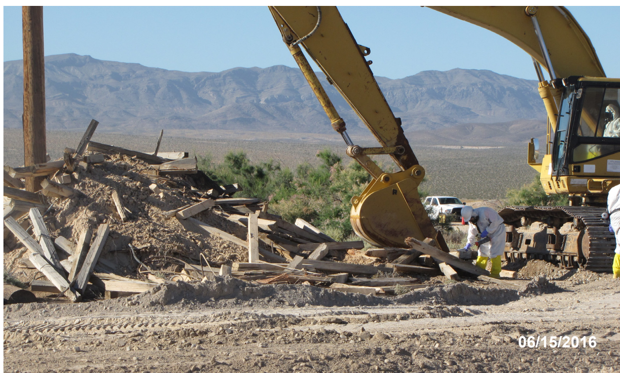
Figure 2-4 Removal of Hamilton Soil/Debris Pile
