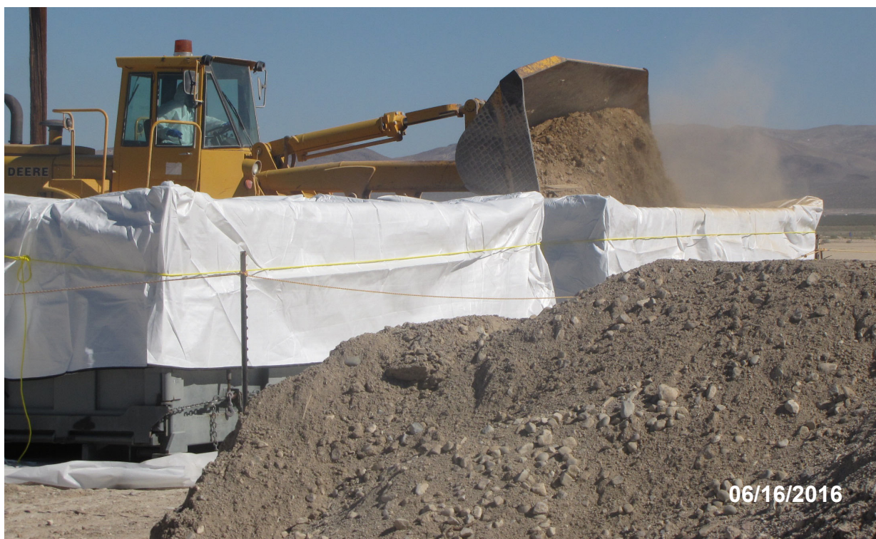
Figure 2-8 Waste Packaging of Soil/Debris Pile Material
