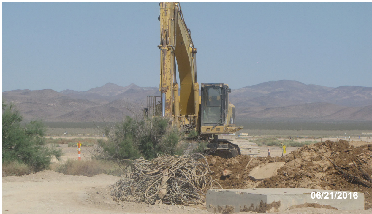
Figure 2-6 Removal of Hamilton Soil/Debris Pile
