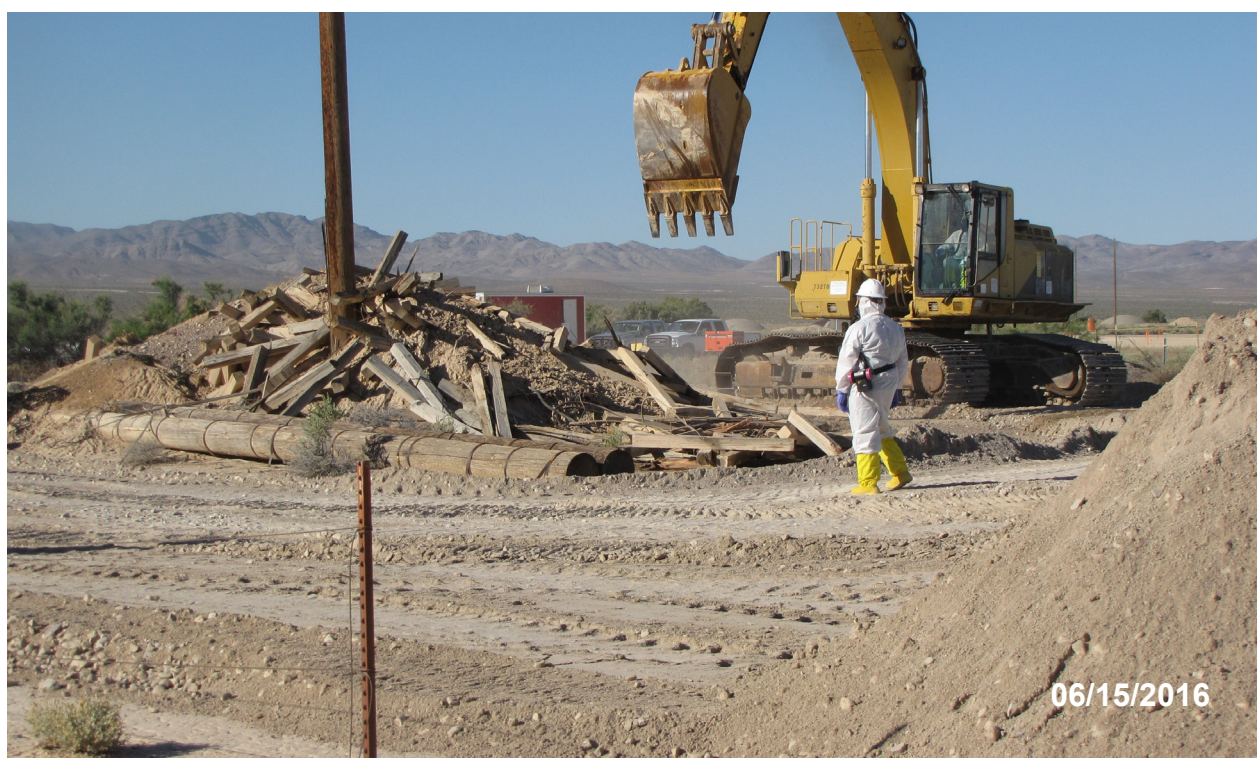
Figure 2-3 Hamilton Site at Beginning of Soil/Debris Pile Removal
