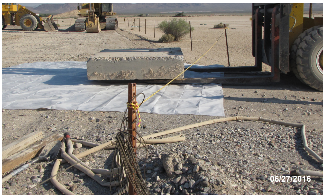
Figure 2-10 Waste Management of Concrete Slab
