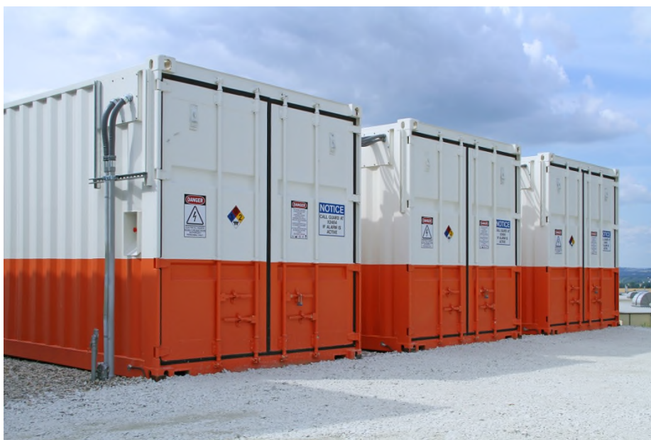
Figure 5. One string of Containerized UltraBattery® System (CUBS)
