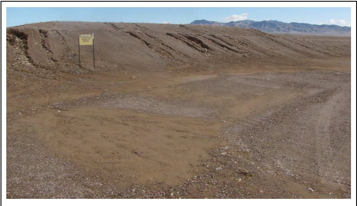
Figure 1-1 Example of Runnels on Slope of South Landfill Cover, Looking East (10/19/2015)
