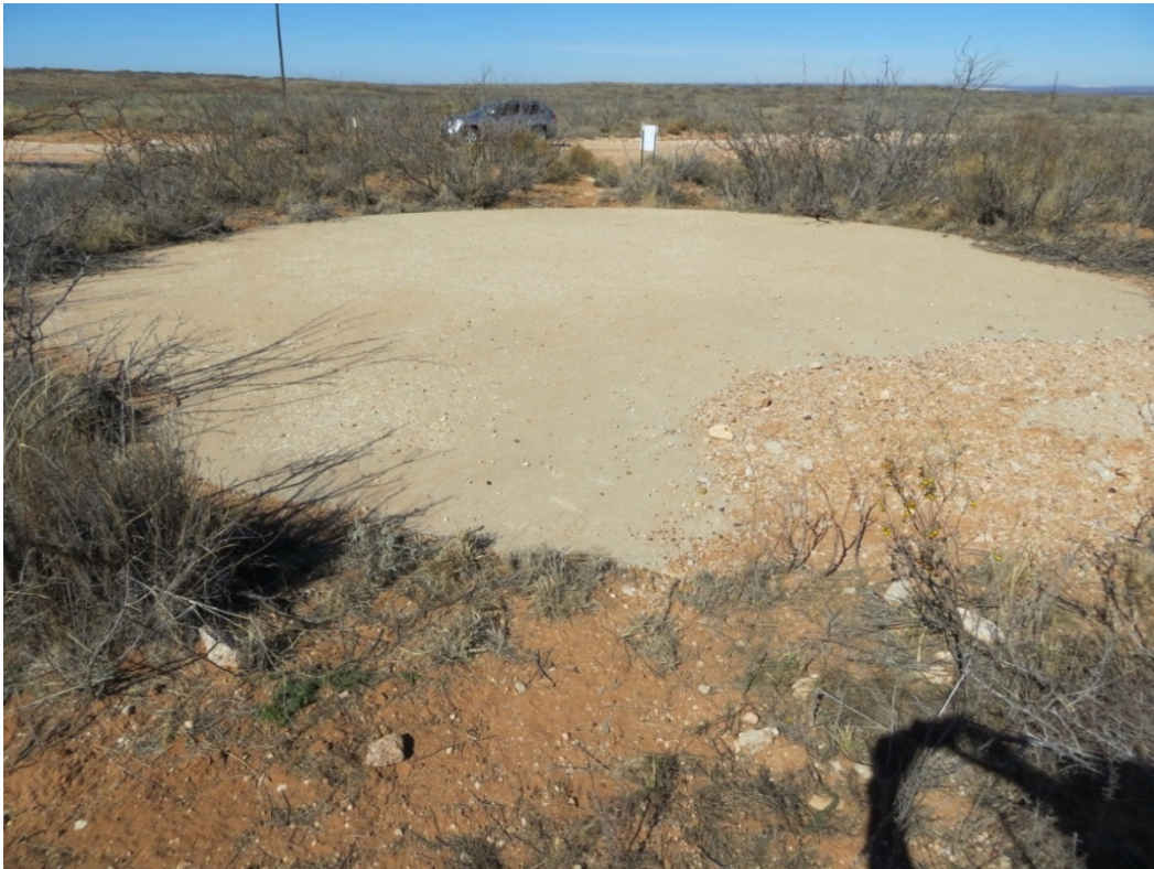
Photo showing the concrete cap that covers the Gnome emplacement shaft.
