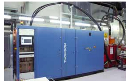
(b) Thomson pulse-step modulator in the MTF hall
