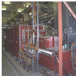
(a) Bouncer-type modulator
