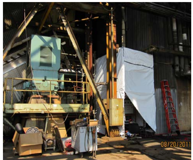
Figure 2-7. Pilot unit inside the tent during field testing
