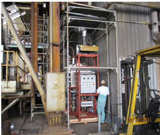
Figure 2-6. Installation of the pilot unit in the field
