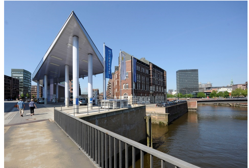
Existing dockside hydrogen station in Hamburg, Germany
