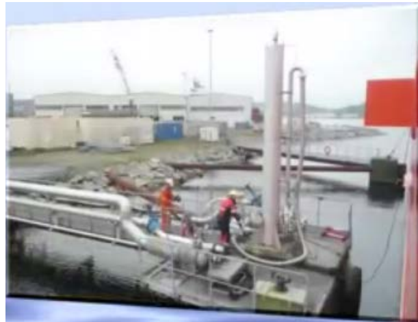
(2) Piping and connecting the fueling arm
