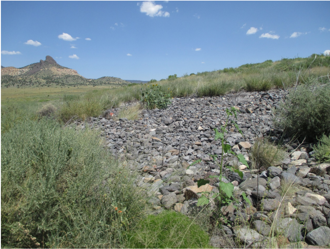
BAR 8/2015. PL-6. Rock-armored slope of containment dam.
