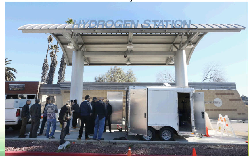
Hydrogen Fueling Infrastructure Research Station Technology
