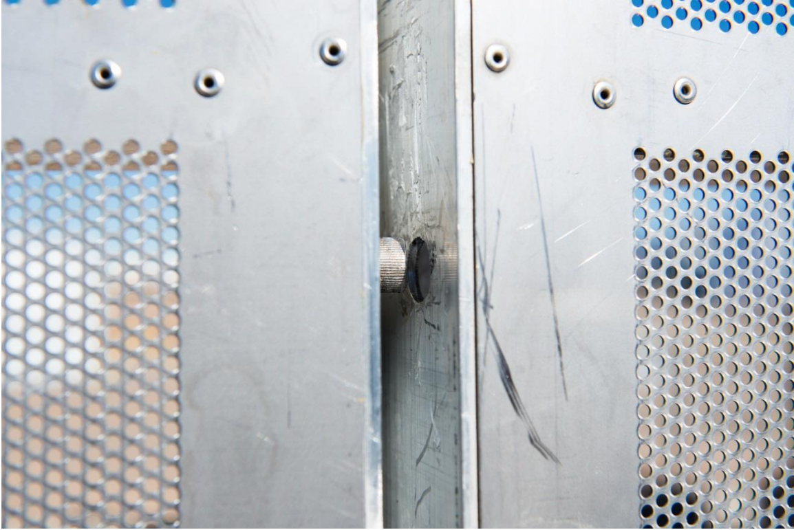
Figure 25 Alignment pin used for adjoining two adjacent straight sections (cont'd.)
