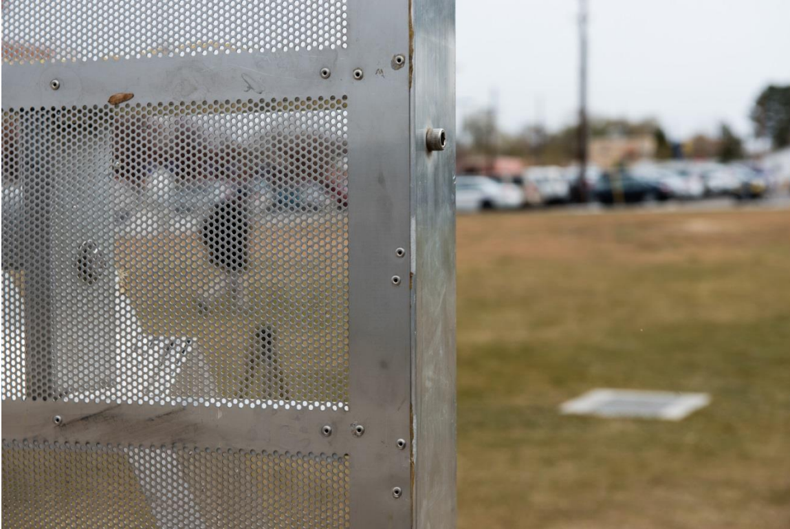
Figure 24 Alignment pin used for adjoining two adjacent straight sections
