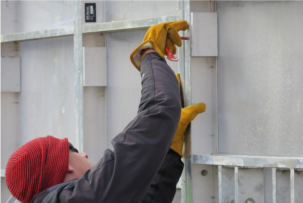
Figure 18 Deployment team member latching a quick lock using one of the hex wrench tools provided
