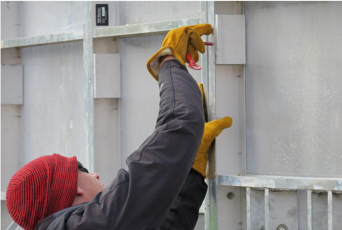
Figure 27 Deployment team member using the hex wrench to latch the quick lock between two uprights
