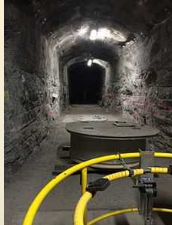
Demonstration tunnel in Olkiluoto
