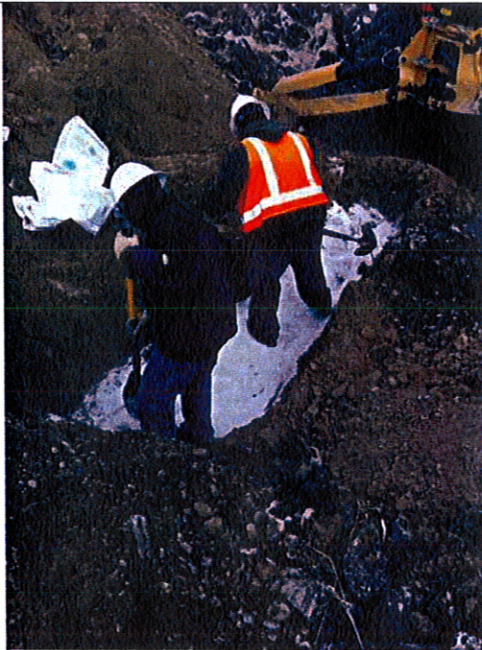
YP personnel Kyle Clemens and Ken Jamison backfilling TP-1 with powdered Bentonite.
