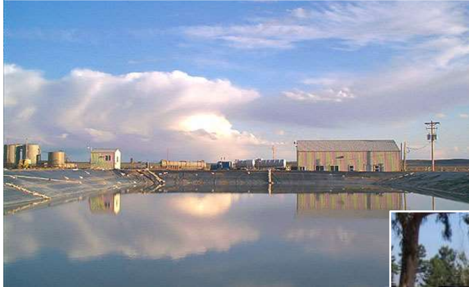
Evaporation pond for produced water
