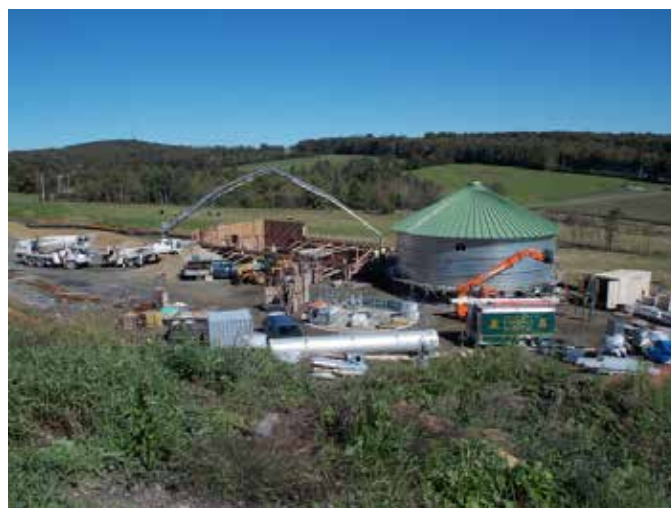
Anaerobic digestion tank is wrapped with Pex tubing to insulate in September 2013.
