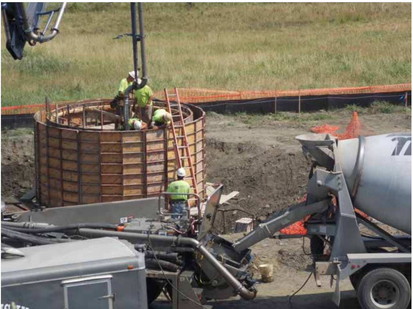
Concrete wall for the liquid effluent tank were built in the last week August 2013.
