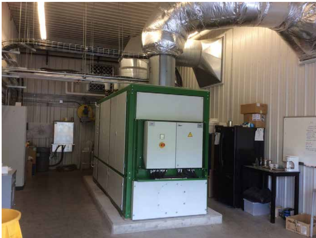
The heat in genset exhaust is captured for reuse.
