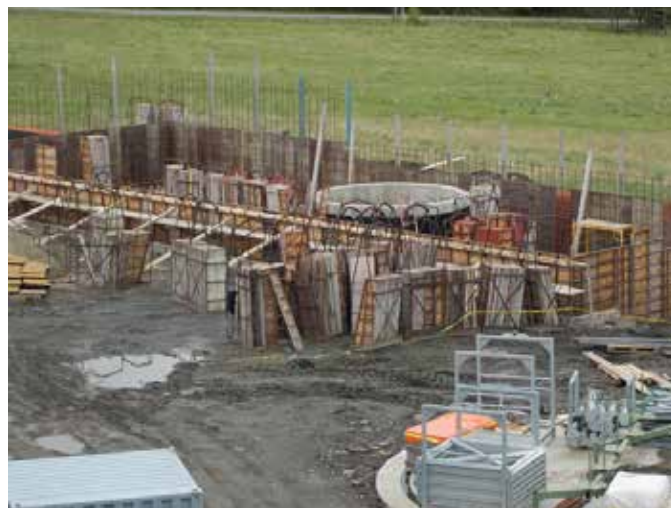
Concrete is poured for the three feedstock tanks.
