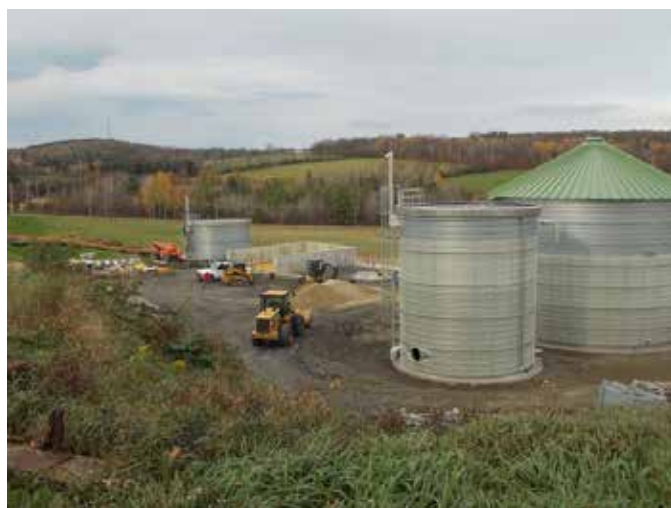
Anaerobic digestion tank and hydrolysis tank under construction.
