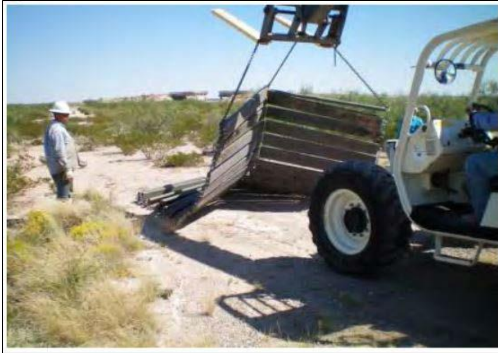
Figure 5: Installation of rollout panels.
