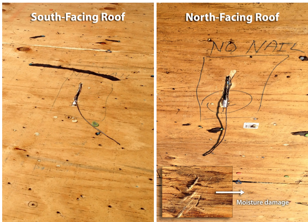
Fig. 7. Condition of the ½-in plywood deck after 2 years of exposure. Replacement shingles and underlayment replaced Feb 2016.
