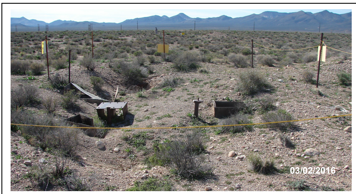
Figure 2-7 SG2: CAS 02-99-12 U2af (Kennebec) Surface Rad-Chem Piping, Vault Area Note: Photograph looking north.
