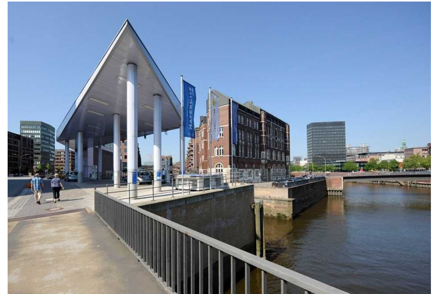
Existing dockside hydrogen station in Hamburg, Germany
