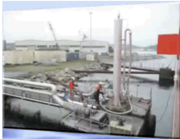
(2) Piping and connecting the fueling arm
