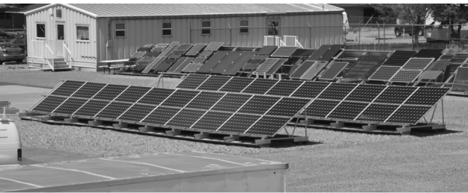
Fig. 2. The present work performed tests on a 10.8kW e array. The array has four strings that each have 10 modules. The strings are combined prior to entering the inverter. In addition, each of the string's current and voltage are monitored.
