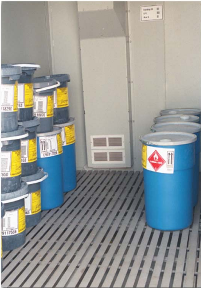
Secondary containment storage area.
