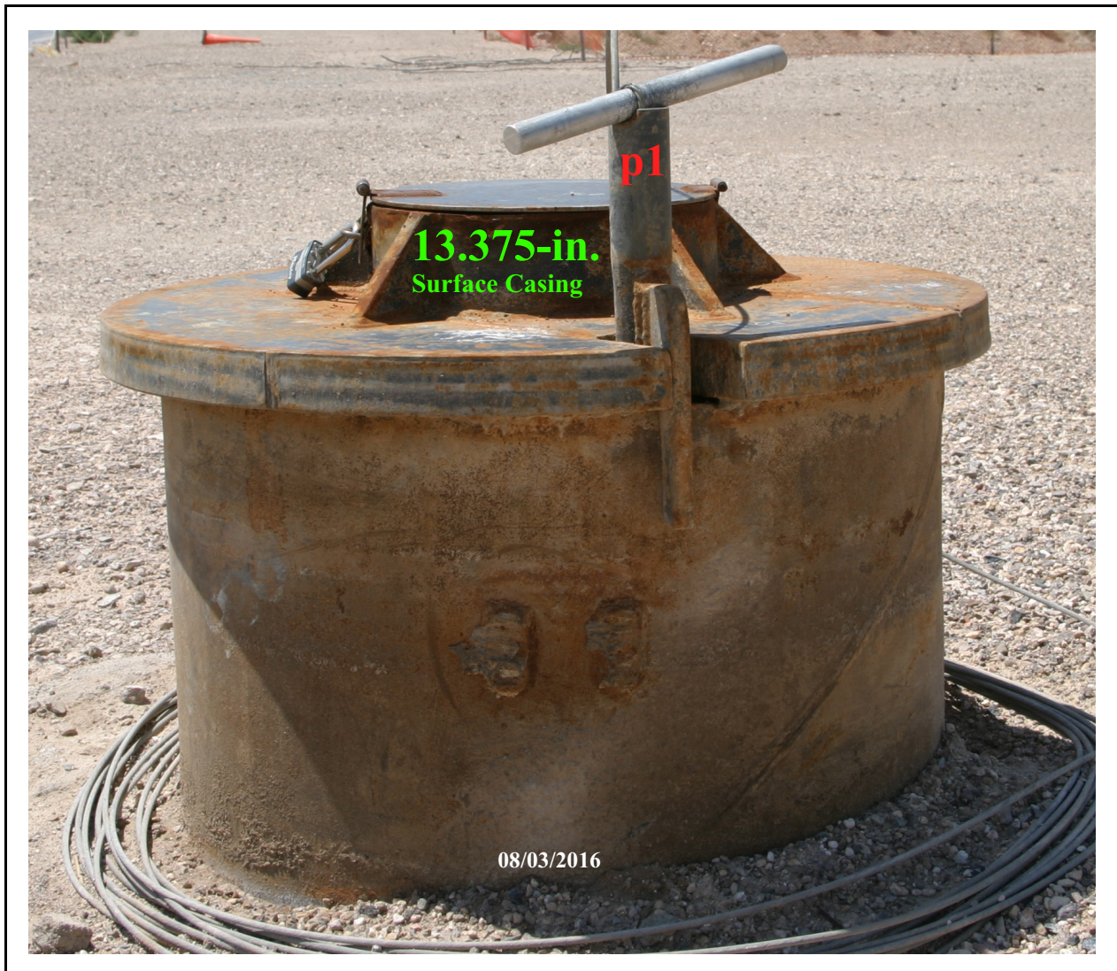
Figure 3-3 Photograph of Well ER-2-2 Wellhead
