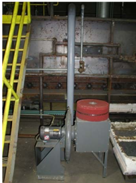
Figure 13. Blower for conveying coal.
