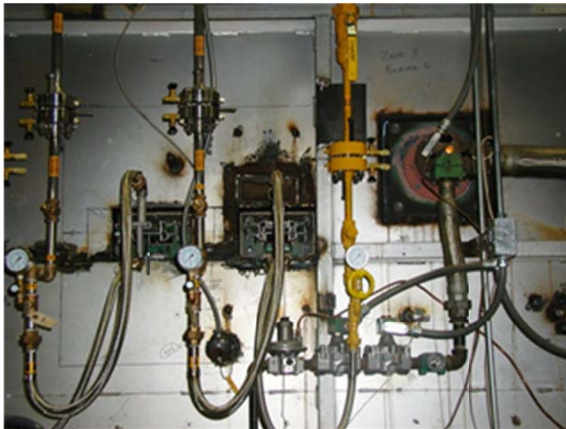
Figure 9. Dual – Combustion system burner arrangement.
