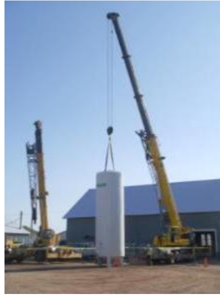
Figure 10. Bulk oxygen tank installation.
