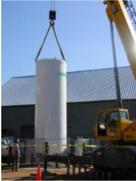
Figure 10. Bulk oxygen tank installation.
