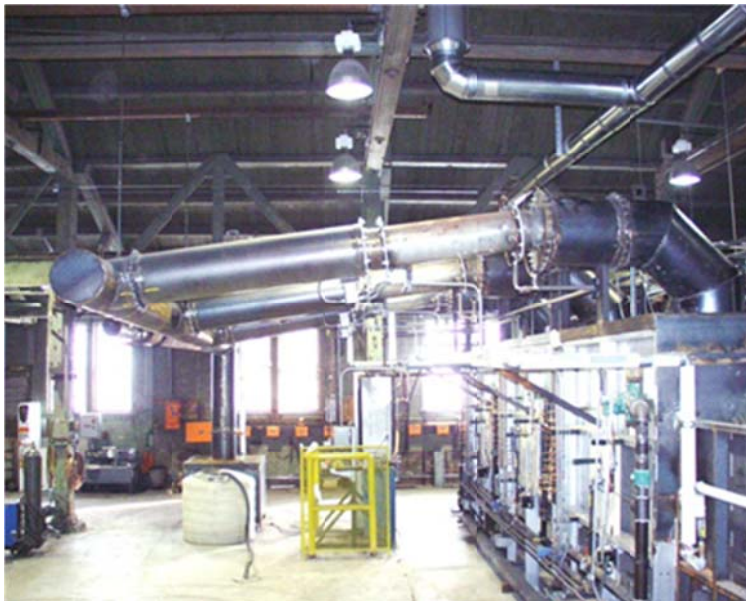
Figure 3. NRRI LHF exhaust duct work.
