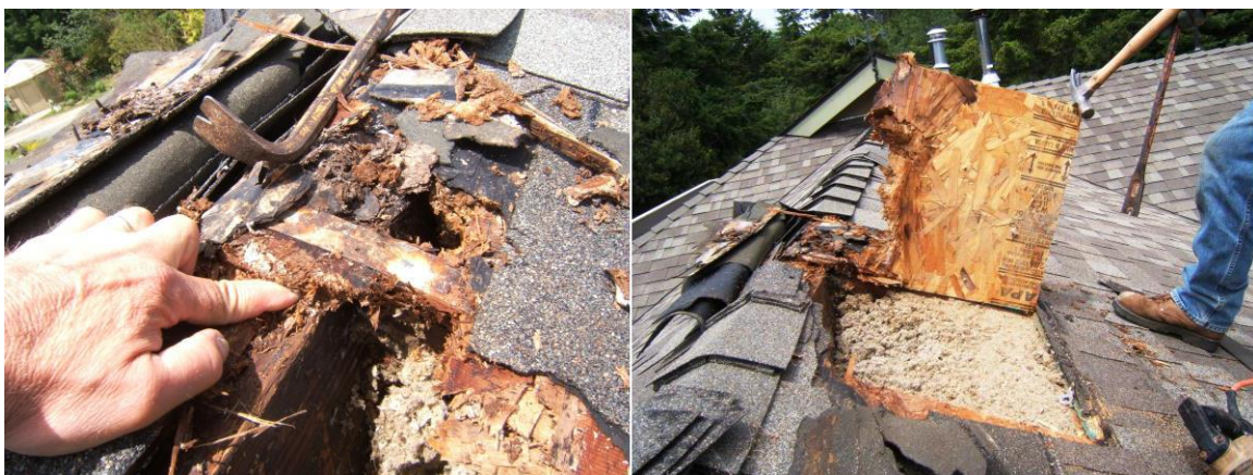
Figure 18 Photographs of deconstruction of a sealed and insulated attic assembly with dense pack cellulose on a home in Northern California that had experienced water dripping at the roof ridge
