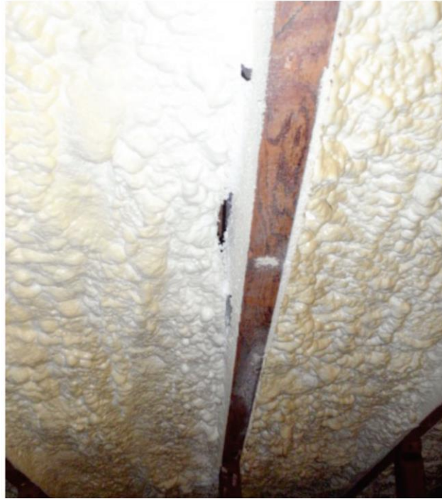
Figure 7 Example image of closed cell SPF delamination from roof framing member. Source: Prahl and Shaffer (2014).
