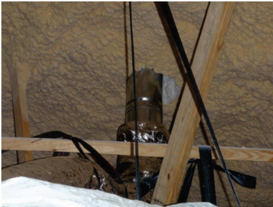
Figure 8 Example picture of gaps surrounding roof vent pipe penetrations. Source: Prahl and Shaffer (2014).
