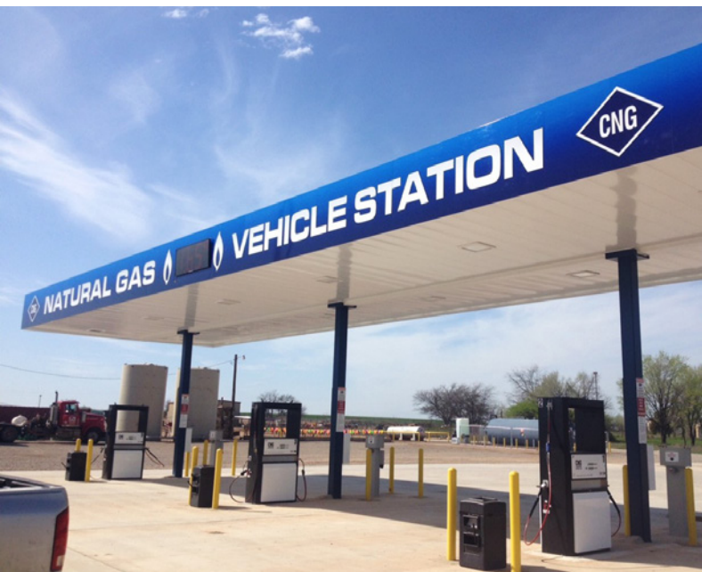
Publicly accessible compressed natural gas fueling station along I-35 in Goldsby, Oklahoma. Photo from Eric Pollard, NREL 39374
