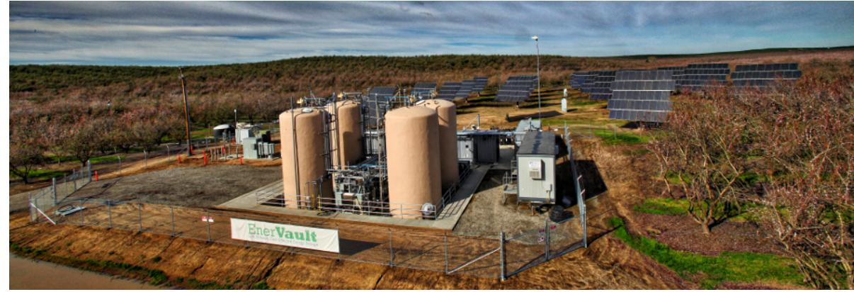
Enervault plant, Turlock, CA. 250kW, 1 MWh.
