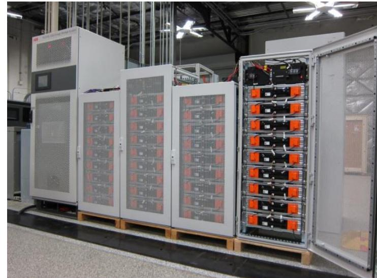
SCE Tehachapi plant, 8MW, 32MWh.
