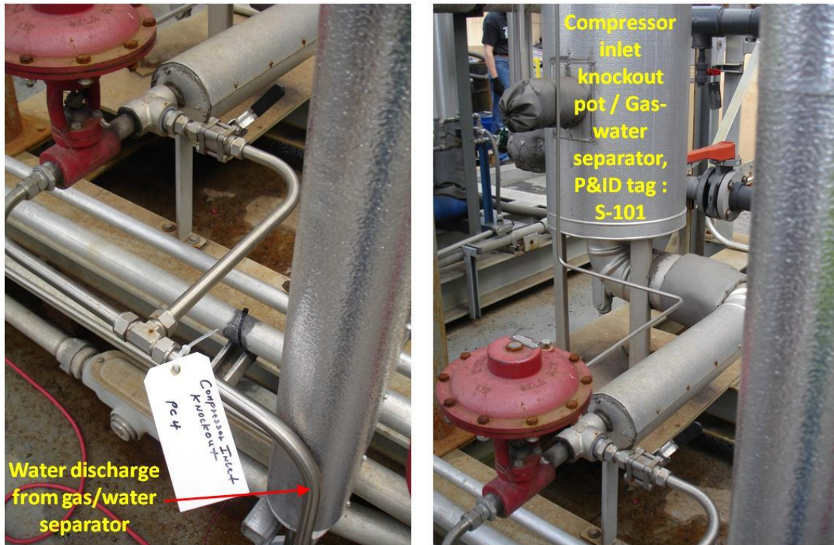
Figure 2-3 Photo of Compressor Inlet Knockout Sampling Location
