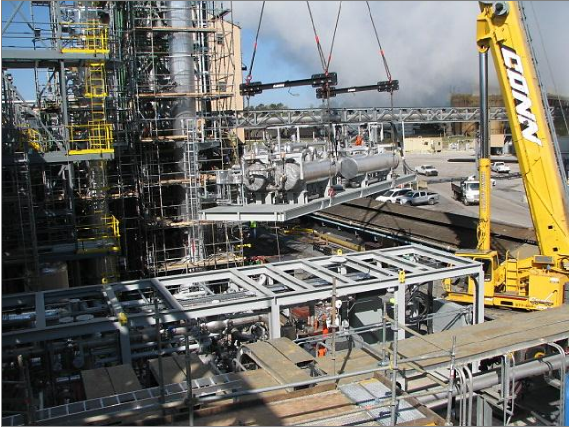
Figure 4.8. A crane lowers the upper level of the 20 TPD system into place during installation.
