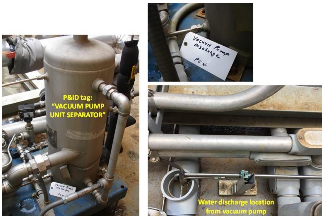
Figure 2-6 Photo of Vacuum Pump Discharge Sampling Location
