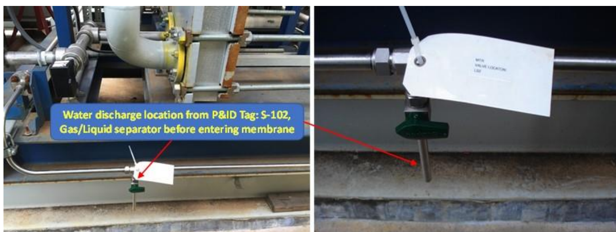
Figure 3-4 Photo of Knockout before Entering Membrane Sampling Location
