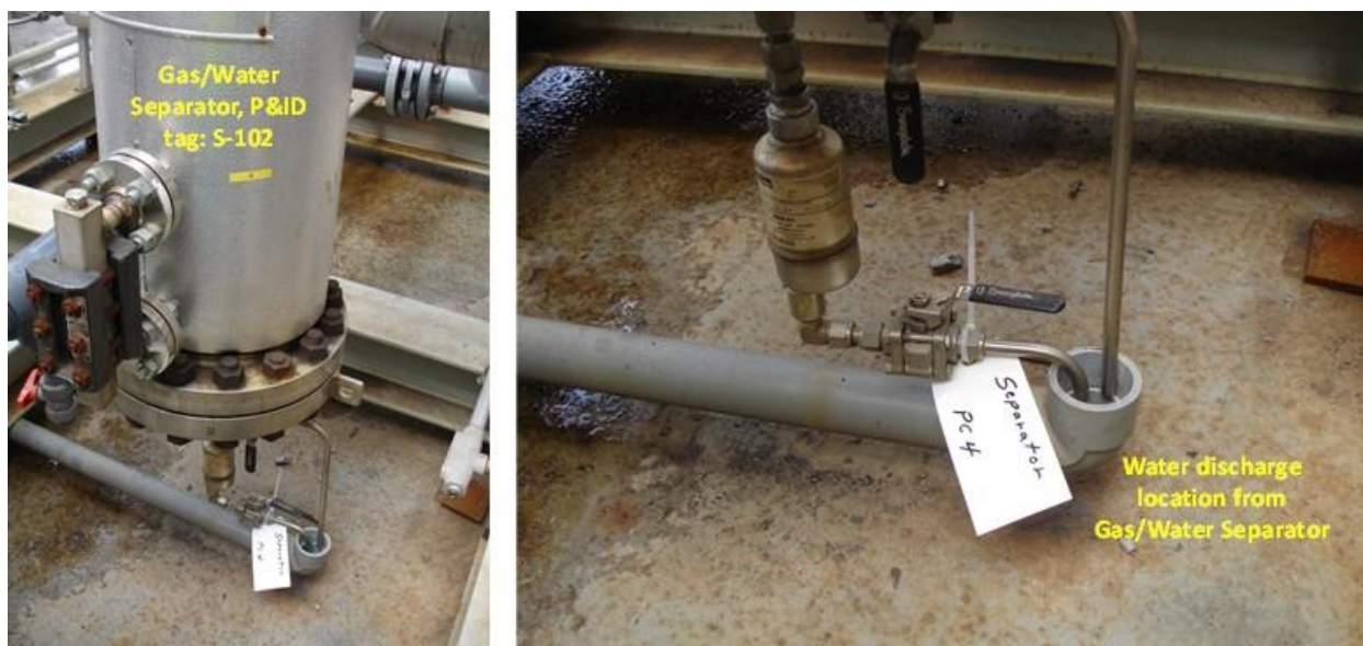
Figure 2-5 Photo of Gas/Water Separator Sampling Location
