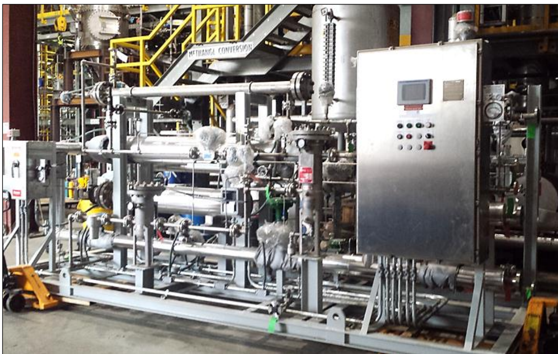
Figure ES 10. A picture of the MTR industrial CO 2 capture test system during installation at the host site in Edmonton.
