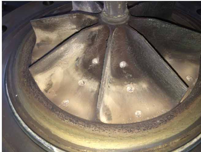
ROG Compressor Impeller Inspection
