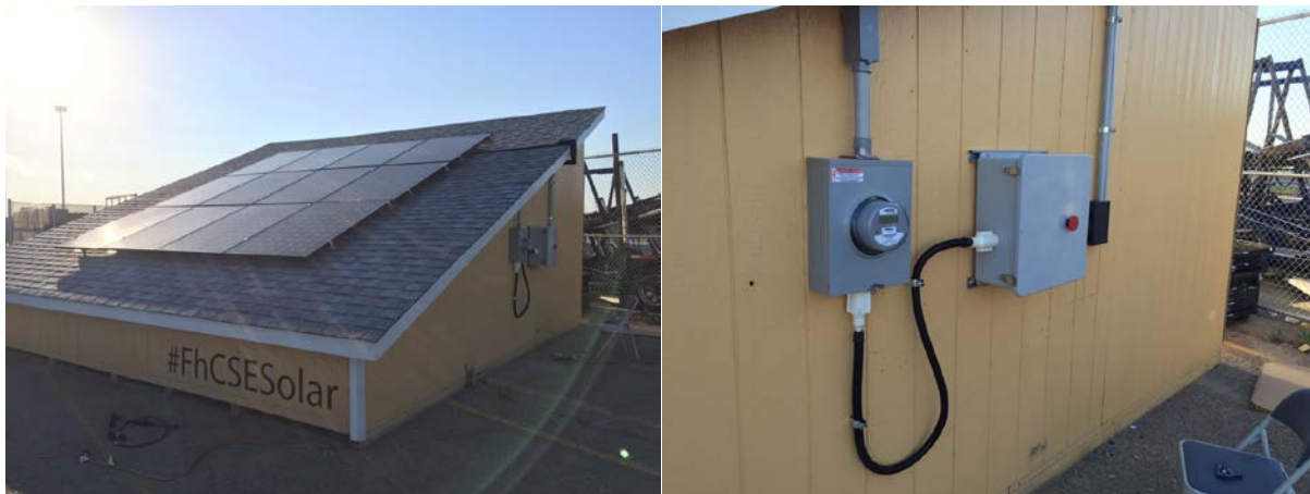
Figure 2-1: SunPower ACPV Plug & Play System Installation
