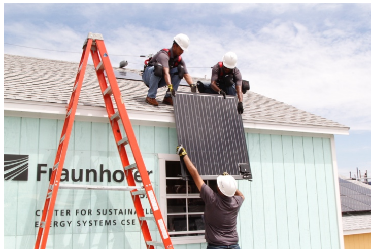
Figure ES-1: The June 2016 demonstration of PnP system installation.
