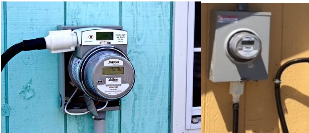
Figure 3-2: Solar Connection Device integrated with a meter collar (left) and meter socket (right)
