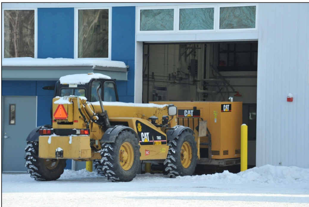
Figure 6. Moving diesel generator into new facility.
