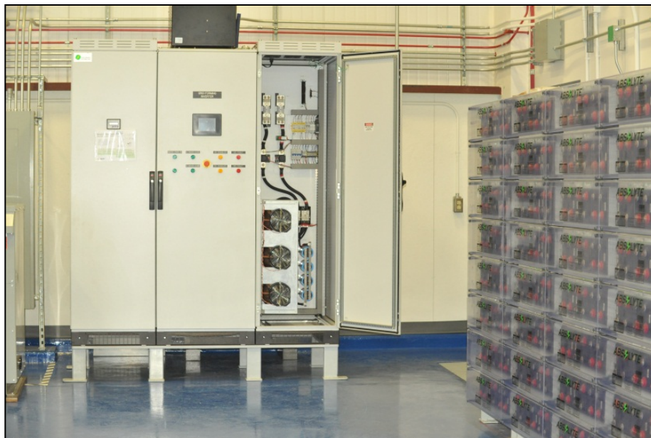
Figure 10. Grid forming inverter undergoing testing at UAF.
