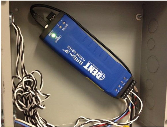
(a) Power meter installed
