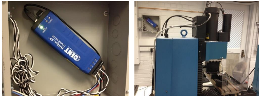
(a) Power meter installed
