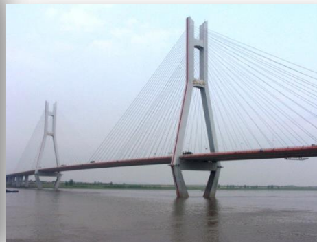
The Wuhan Junshan Bridge over the Yangtze River is covered with 35,000 m 2 (~8.5 acres) of thermal sprayed zinc coating!
